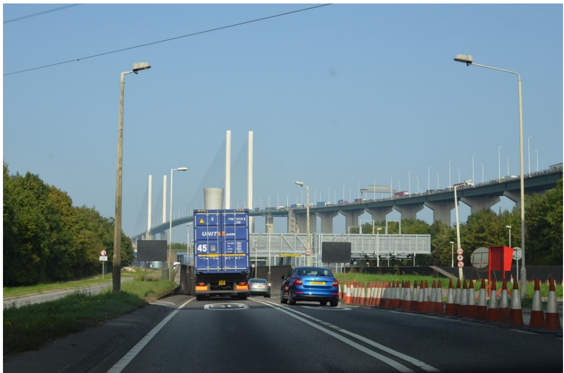
PHOTO 1 - APPROACH TO DARTFORD CROSSING (SOUTH SIDE)
